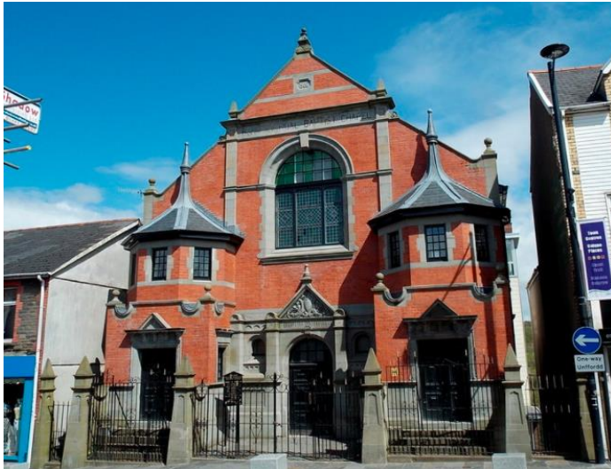
Figure 7: Hanbury Road Baptist Chapel & Schoolrooms, Bargoed
